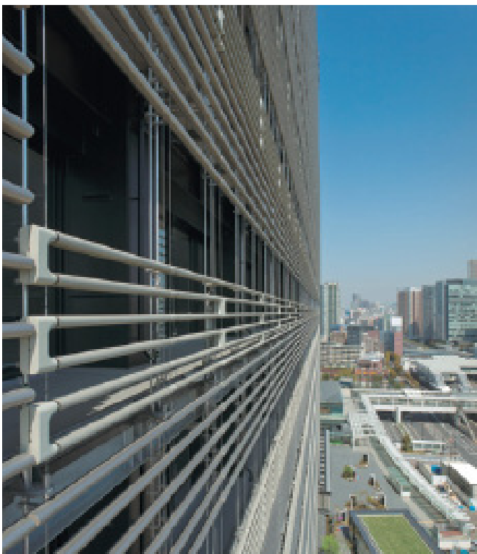
Figure 100: Facade view of the Sony City Osaki building project and the BIOSKIN system (NIKKEN SEKKEI LTD. 2011).
