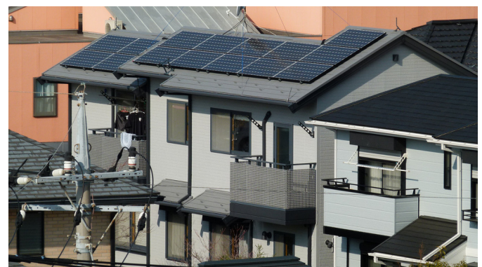
Figure 62: Photovoltaic system on a typical Japanese house (CoCreatr 2011)
