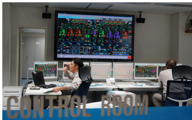
Figure 60: Control room of the Shinjuku DHC plant (m:ci 2013)
